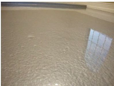
Finished Metallic Floor
